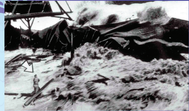
Hilo Harbor, Hawaii, April 1, 1946, Aleutian Islands earthquake. Photo taken from the vessel Brigham Victory of tsunami breaking over Pier 1. The gentleman on the left did not survive. (NOAA)
