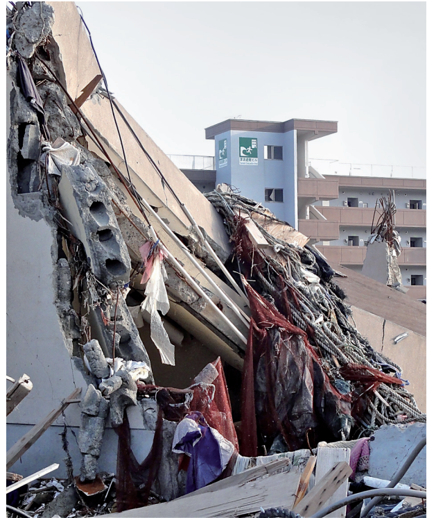
Tall reinforced concrete buildings served as vertical evacuation refuges during the 11 March 2011 Japan tsunami, saving many lives. Minami Sanriku, Japan. Photo courtesy of ITIC.
