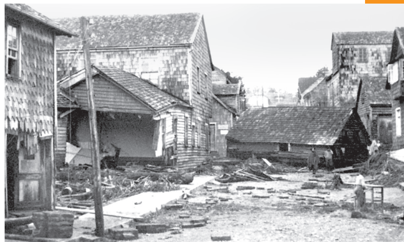
Damage caused by the 22 May 1960 Chilean tsunami. Photo courtesy of Ilustre Municipalidad de Maullin, USGS Circular 1187.
