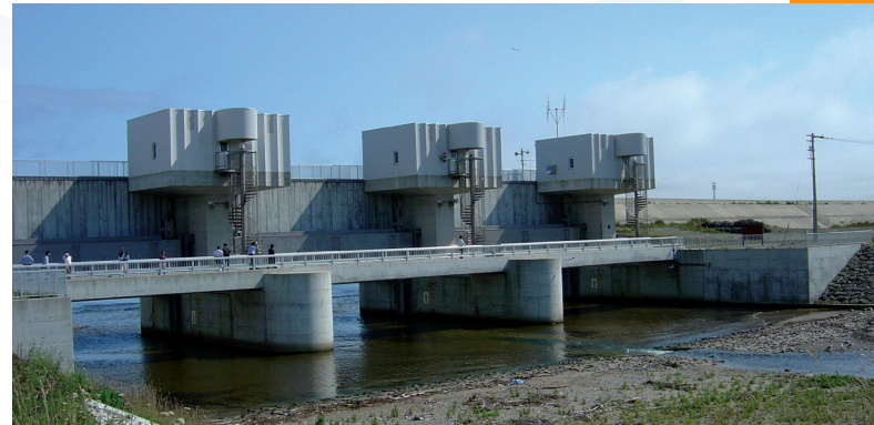
Water gate used to protect against tsunami waves on Okushiri Island, Japan. The gate begins to automatically close within seconds after earthquake shaking triggers its seismic sensors. Photo courtesy of ITIC.
