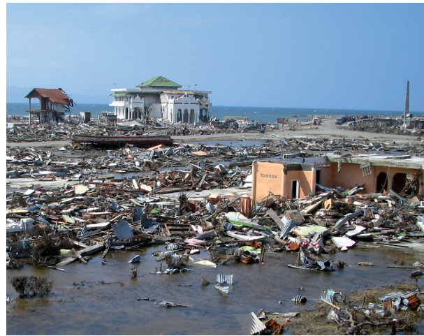
The tsunami of 26 December 2004 destroyed the nearby city of Banda Aceh, Indonesia, leaving only a few structures standing. Photo courtesy of Yuichi Nishimura, Hokkaido University.
